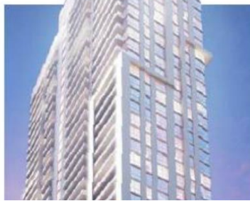
RIGHT: Construction is underway for The Bond at Brickell
