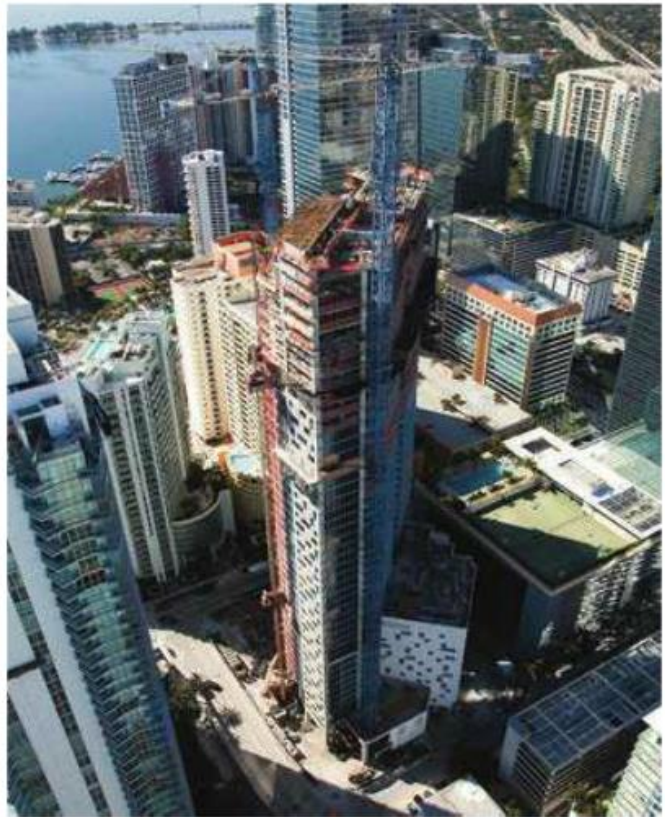
Construction on BrickellHouse
