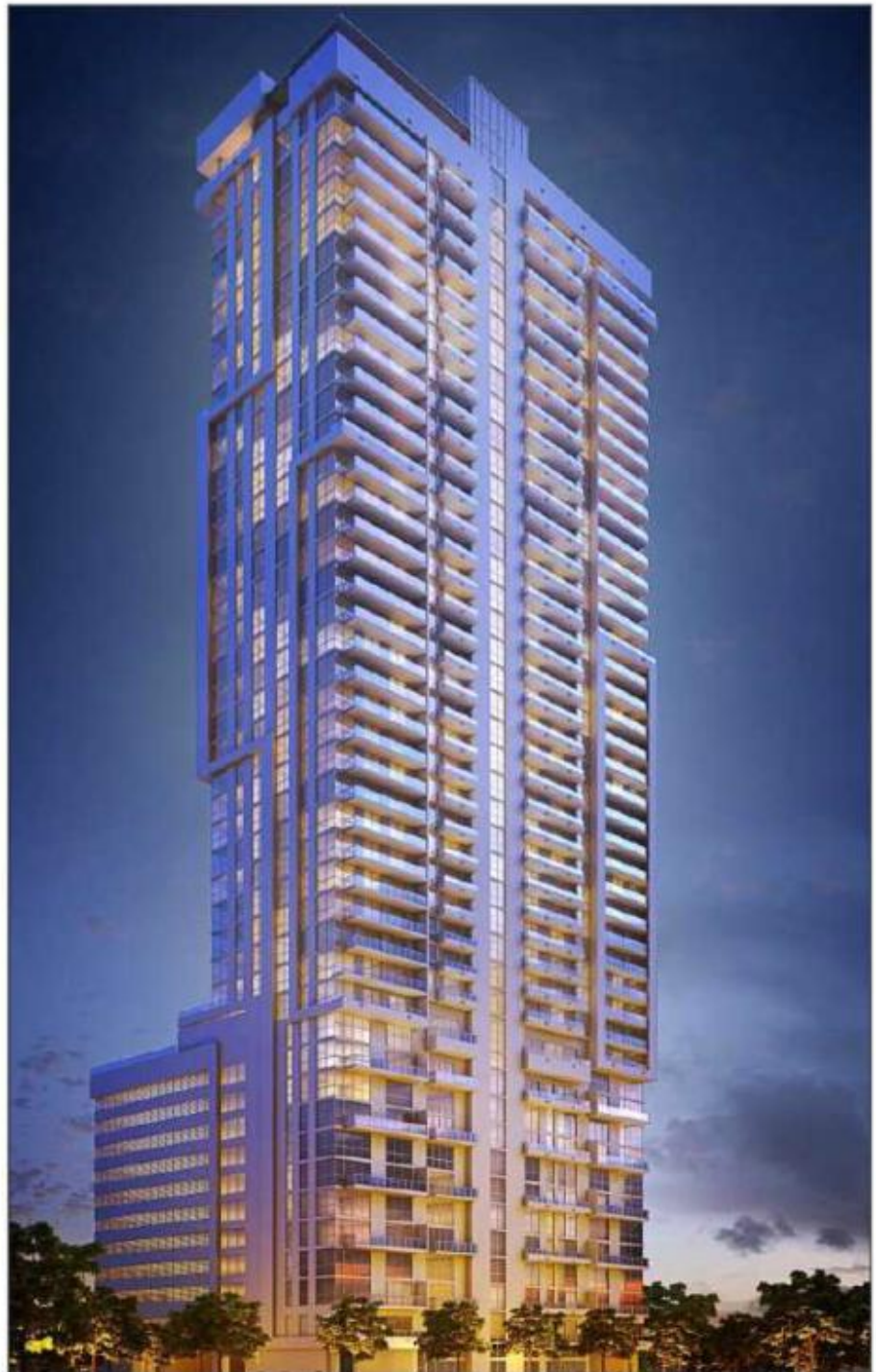
THE BOND: Prices at the condominium project unveiled by Rilea Group will run from about $300,000 to more than $1 million.
